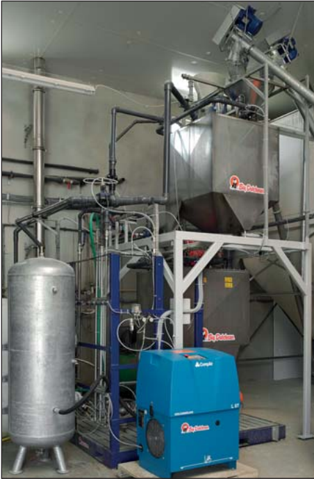
HydroAir-Synchron – this double-tank system supplies large stocks without long waiting times
